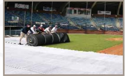
*The 16' x 150' strips of EnkamatPlus are simply rolled out onto the field and held in place with ordinary landscape staples. Total installation time was less than 3 hours.*
