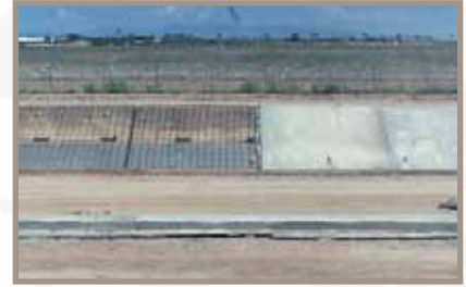
Geotextile fabric holds back concrete.
