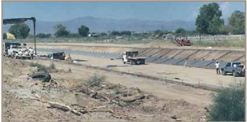
A seven mile stretch of the Agua Fria highway in Phoenix uses Enkadrain instead of aggregate and fabric.
